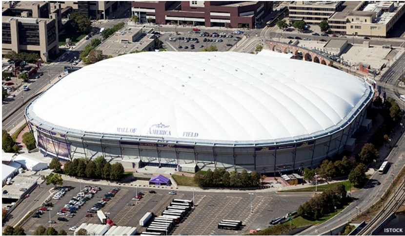
Metrodome, Minneapolis, MN
